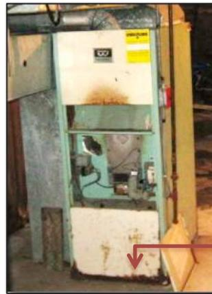
“Moisture from the concrete wicks up through the insulation on the inside of the blower compartment and causes the metal cabinet to rust out.”
